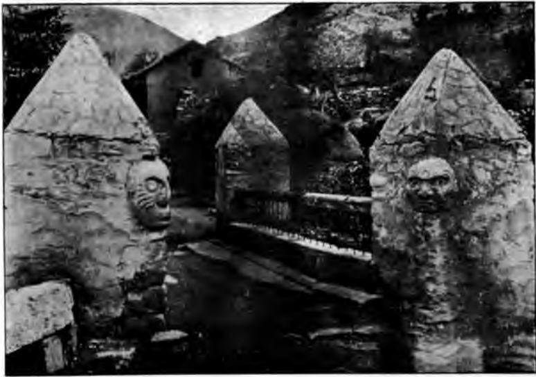
INCA BRIDGE NEAR CHAVIN.
